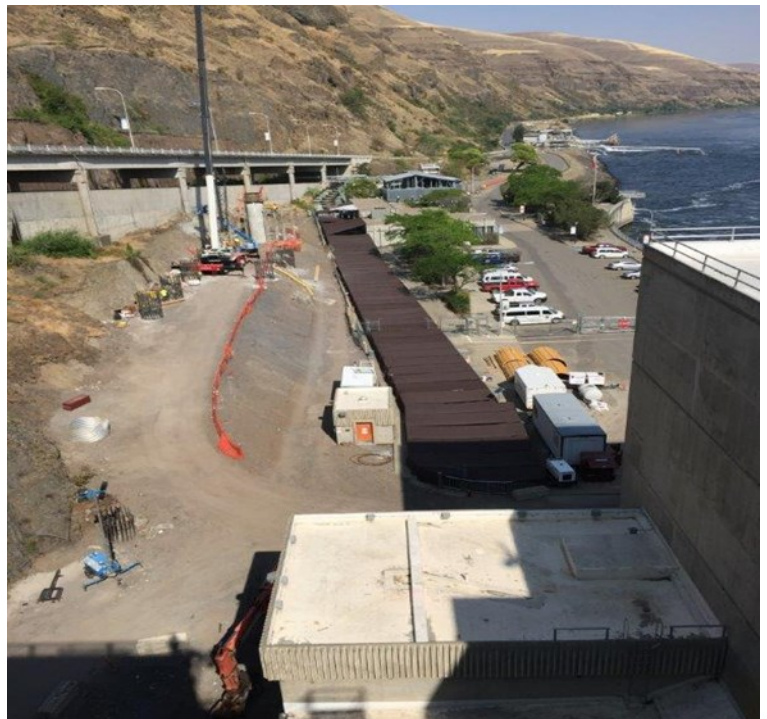
Figure 3. Lower Granite transport flume under construction. July 2015
